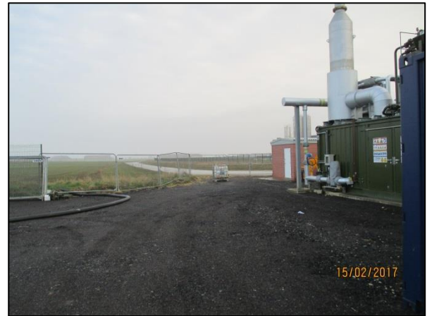
View of site (looking north)
